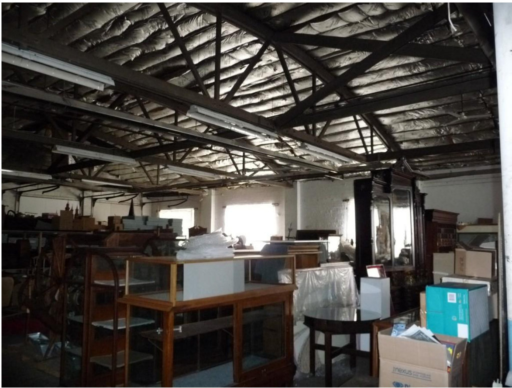
Spray insulation would be applied in between the ceiling joists allowing the bow trusses to remain exposed.
