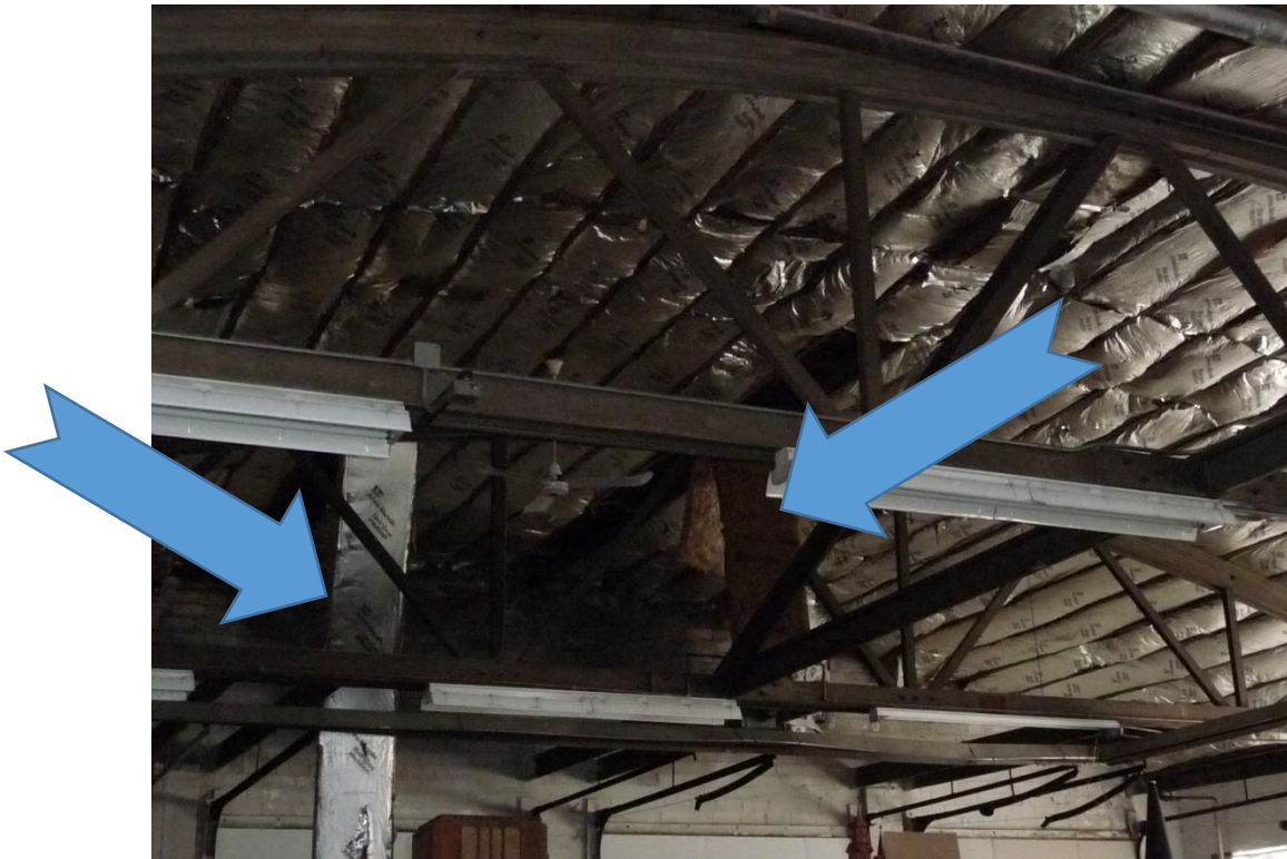
Current insulation falling from the ceiling
