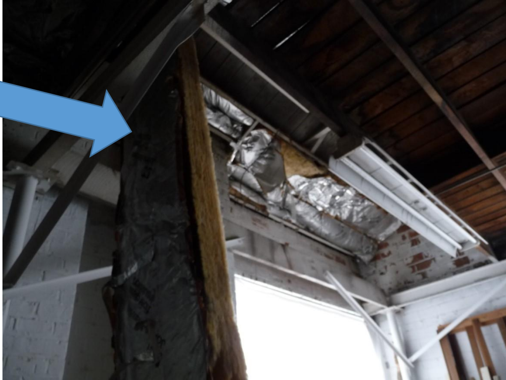
Current insulation falling from the ceiling
