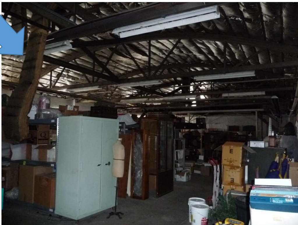
Current insulation falling from the ceiling
